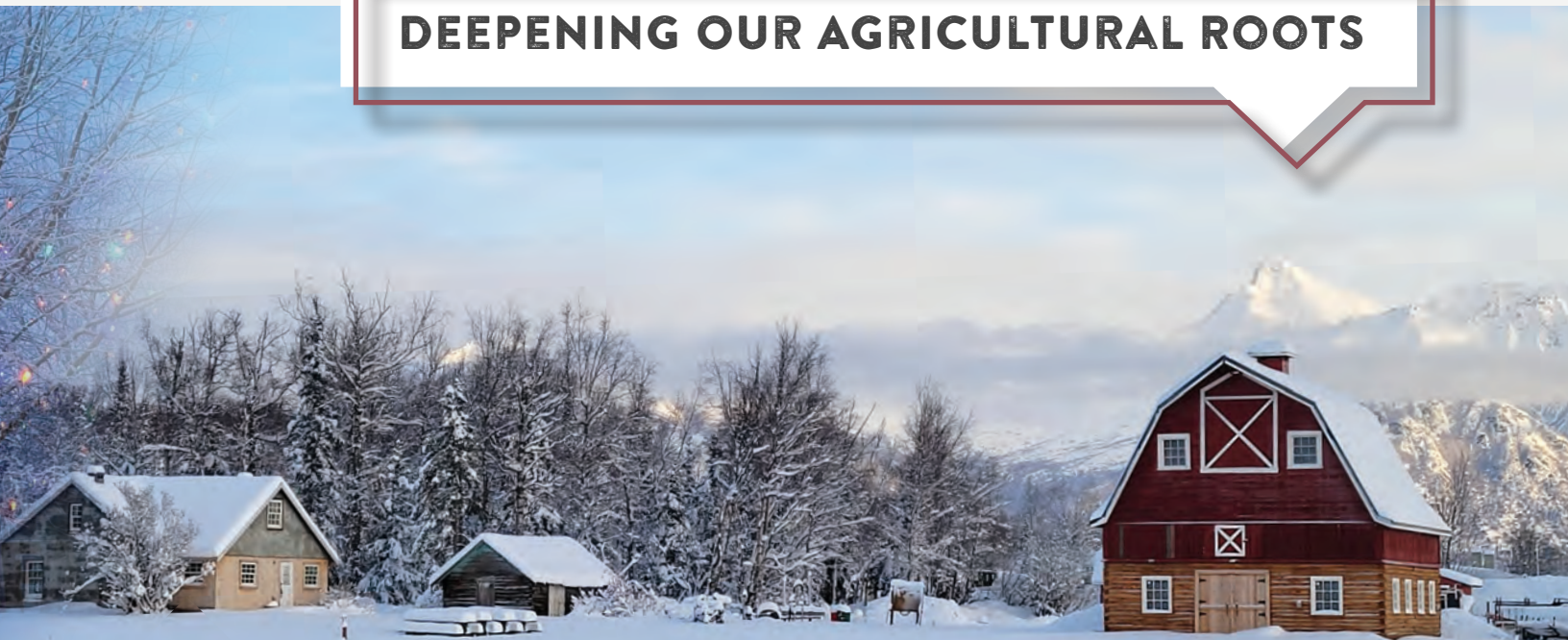
Newly renovated Sjodin Barn was built in 1936 and relocated to Rebarcchek Farm in 2021.
